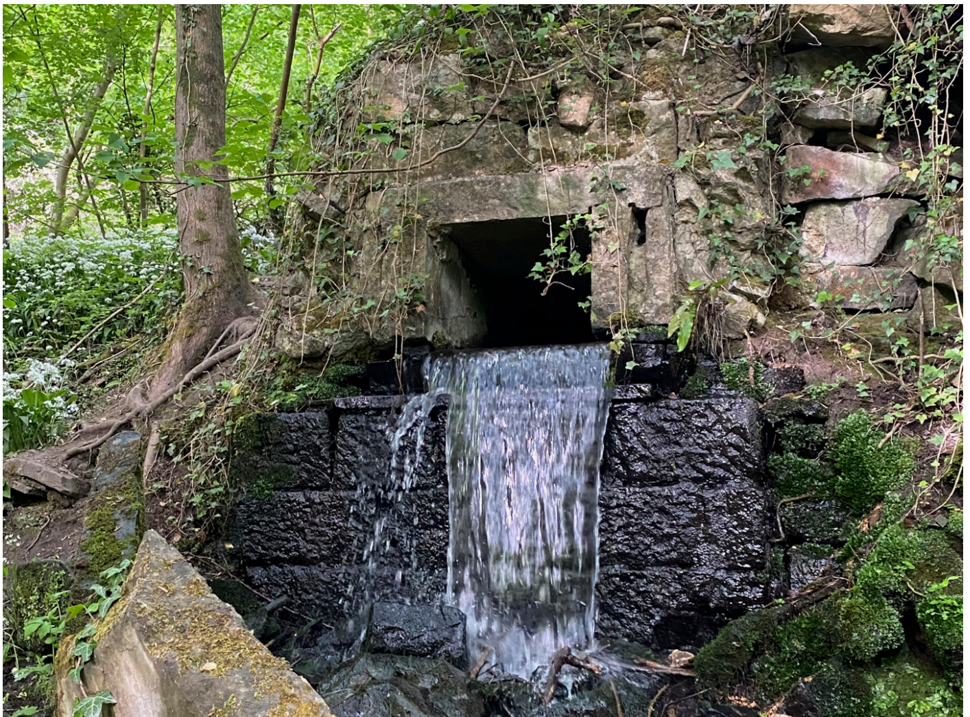
Figure 6. Sluice in the retaining wall, which housed the water wheel(s)
